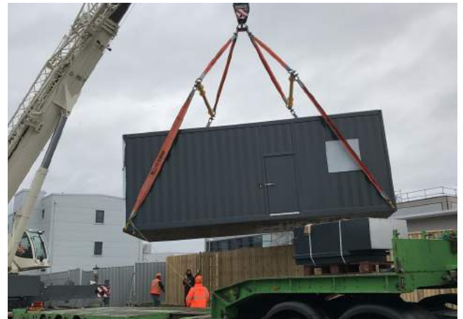
The acoustic enclosure is lifted into position on-site
